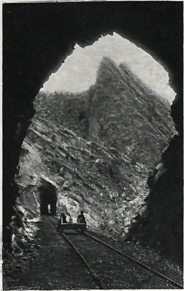
TUNNEL ON THE ROCKIES.
