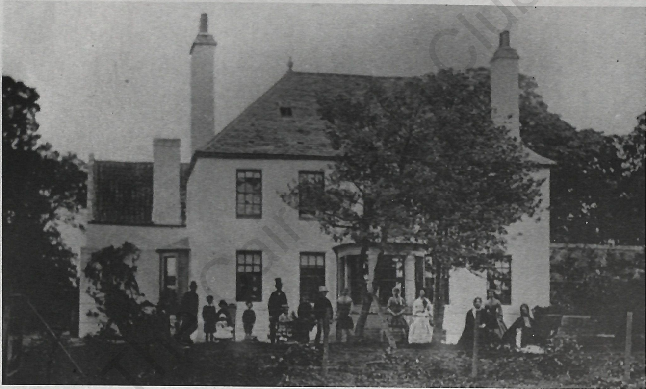
Figure 1 Fountainhall House, Aberdeen, around 1880, before Blenheim Place was built.
