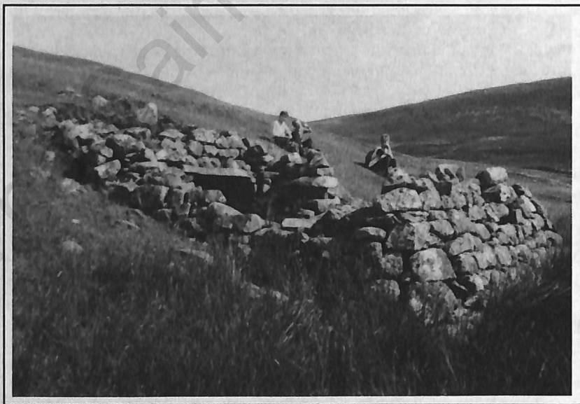
Lime kiln at Dalnafae in Glen Ey.
