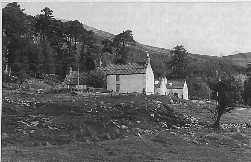
Allanaquoich farmhouse and steading showing the asbestos roofing which has now been removed
