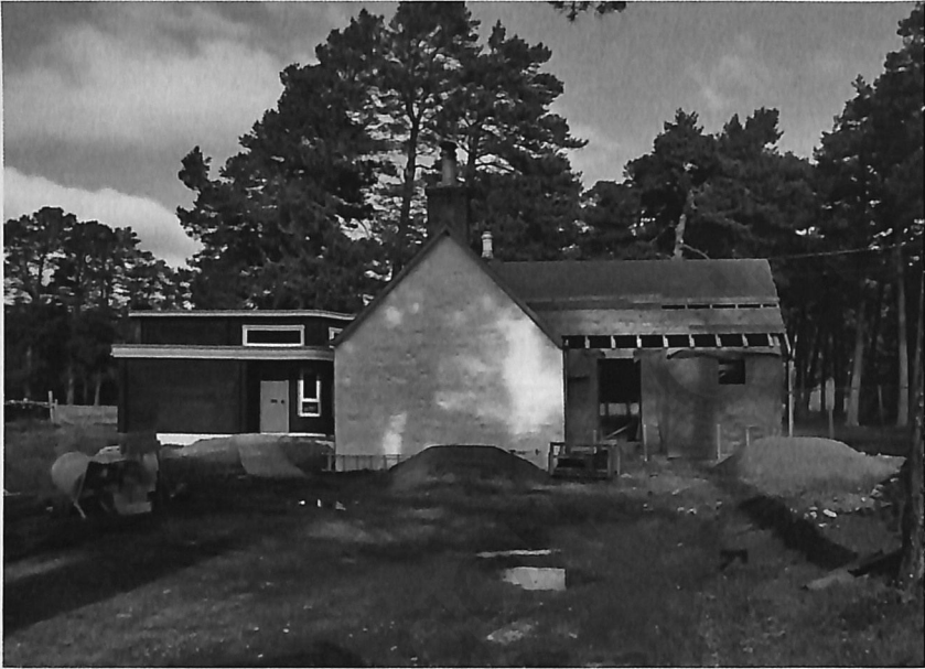
Rebuilding in Progress
