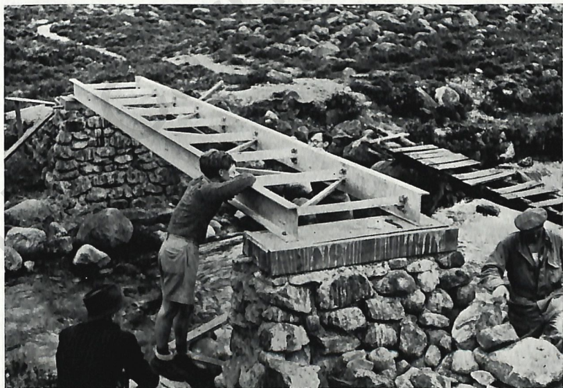
LUIBEG BRIDGE UNDER CONSTRUCTION
