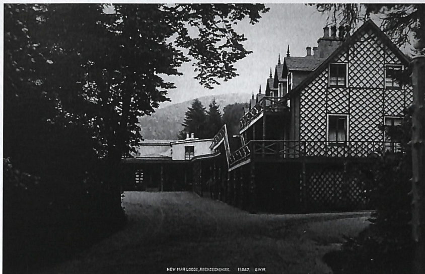
Figure 2 New Mar Lodge before 1893. Photograph by George Washington Wilson.
