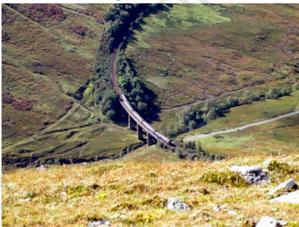
Fig 4. Glen Coralan Viaduct/West Highland Line. Photo Brian Davey
