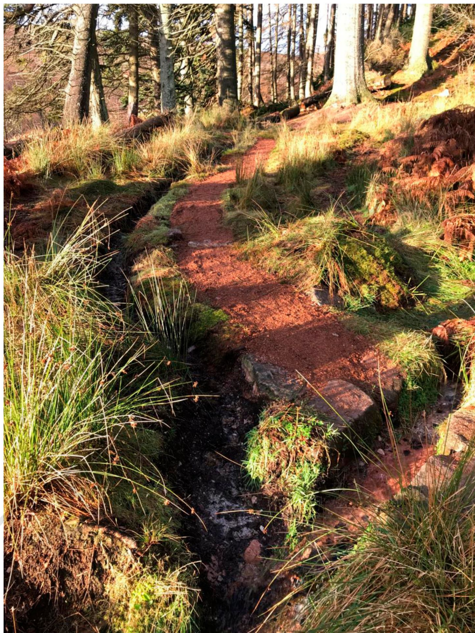
3 Cross Drain and ditching (funded by the Club)
