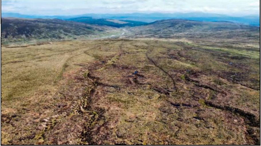
Aerial view of work in the Cairngorms
