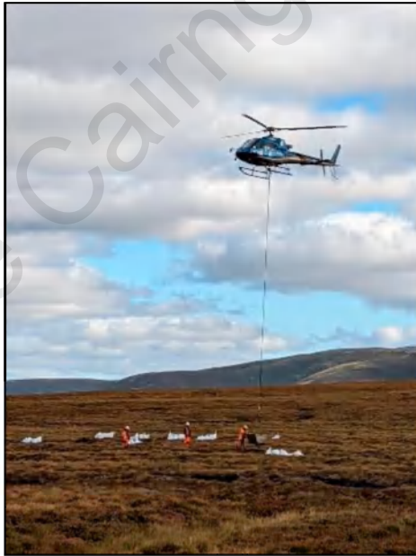
Lifting heavy materials into inaccessible spots Photo credit Matt Watson
