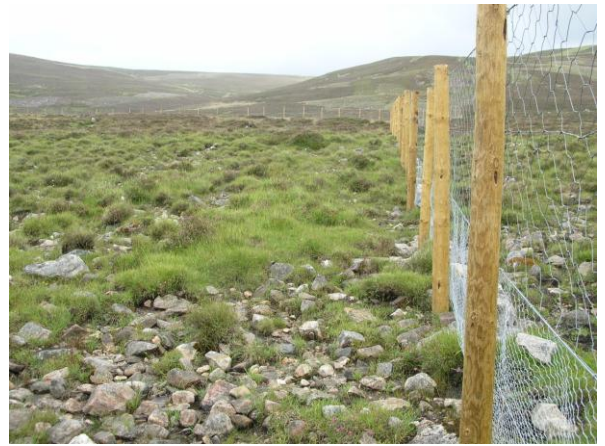
Corner D: view uphill along new fence line, Aug 2013
