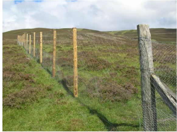
Corner A: looking up new fence line, Aug 2013
